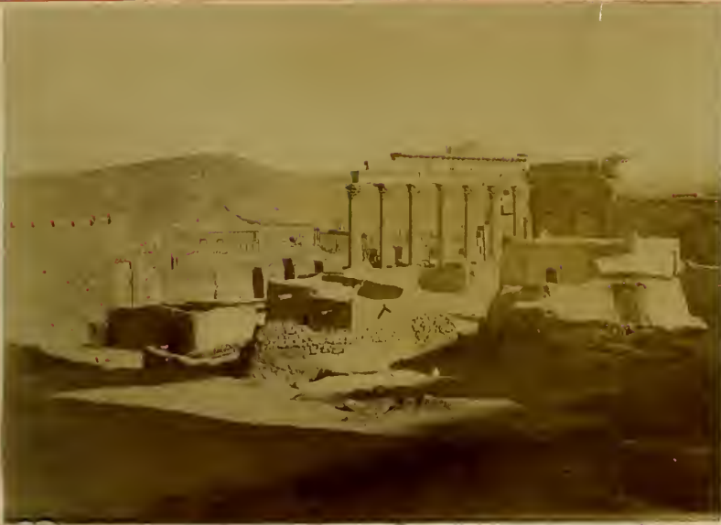
Temple of the Sun enclosure, toward the N.W.
