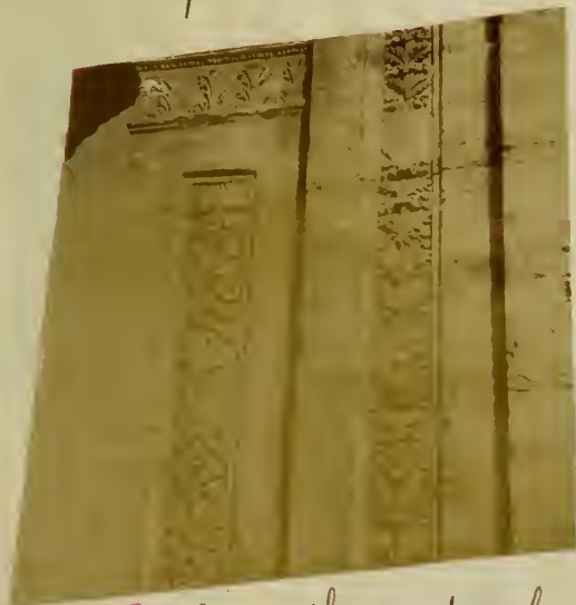
Panels in the great arch.
