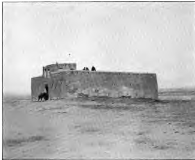
1. THE WELL OF ASRA. 2. GUARD HOUSE AT AIN EL BEDA.
